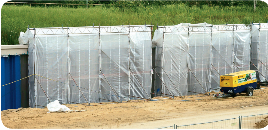
The coatings are applied section by section over 300 m.
